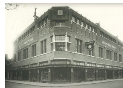
V&D-gebouw na opening in 1934.
