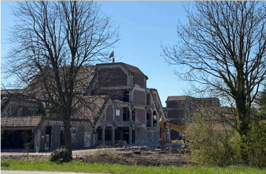
Begin 2026 was de sloop in volle gang. Foto: M. Alphenaar
